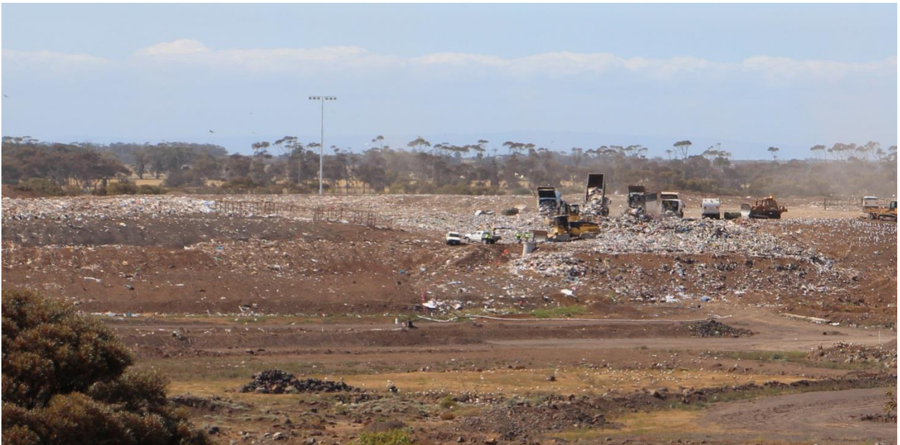
Tipping face greater than 25m x 25m – note the uncovered waste adjoining the tipping face
