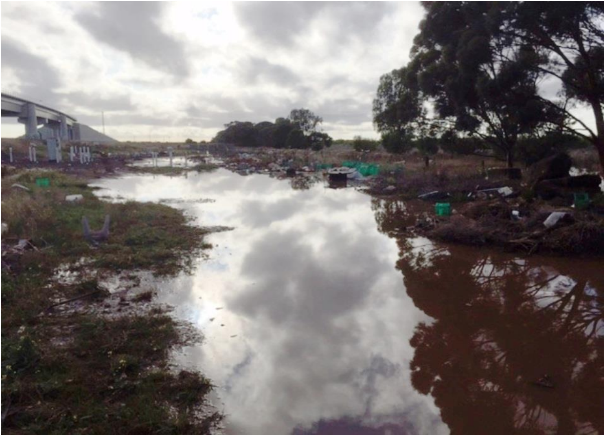
Flooding adjacent to landfill site 2017
