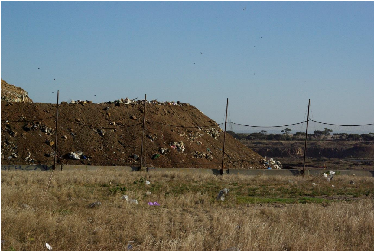
Waste mountain showing steep batter and visible waste
